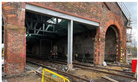
Work in progress to restore the 1861 Whessoe Road engine shed, note the new roof trusses in place and preparations to pour the concrete floor.
